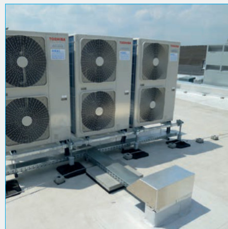
Modular air conditioning solutions with redundant production of refrigeration
