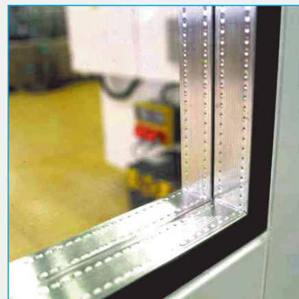
Glazing meeting GMP standards with continuous silicone joint
